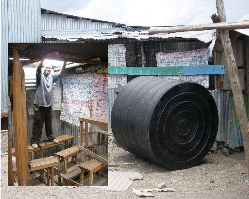
St. Tim Renovations
